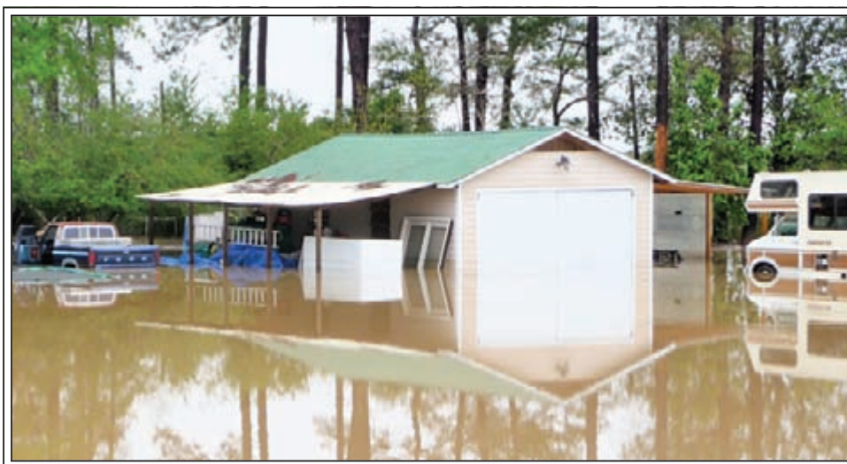
Home and buildings on SR 45 south in Colquitt get flooded out.
